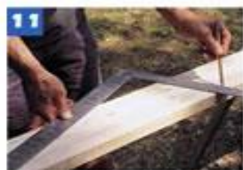
11 To find the rafter cutting angle, align the 5- and 12-in. marks on the framing square's legs with the edge of the rafter stock.
