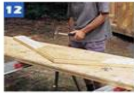
12 To find the rafter cutting angle, align the 5- and 12-in. marks on the framing square's legs with the edge of the rafter stock.
